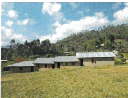
Newly roofed classroom
