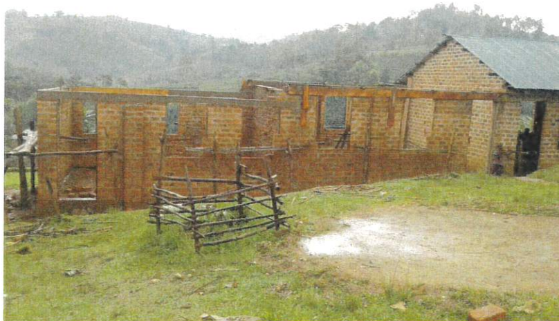
The latest photo – taken a week after construction started!
